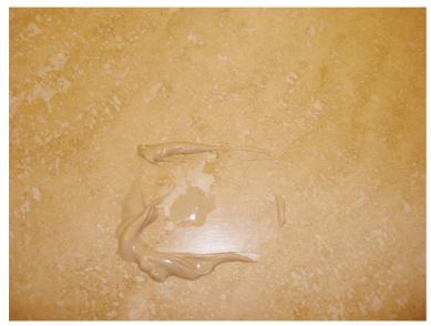
**STEP 6.**Using a flat sided filling or putty knife push the filler in to the affected area to ensure all the cavity is filled.
