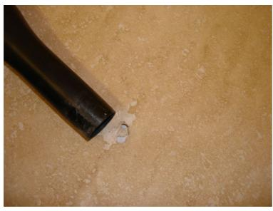
**STEP 1.**Remove any remaining loose filler and dust, the easiest way is to use a hover to thoroughly clean out the affected area.
