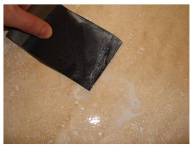
**STEP 10.**Using a fine grit wet and dry sheet, apply a small amount of water to the area where the filler is and rub the filler to remove the excess product until you get to the desired level / finish.
