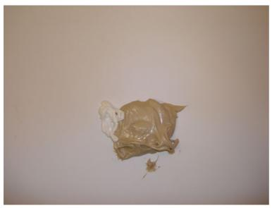
**STEP 2.**Take out only the amount of filler required to fill the immediate effected are. The filler is mixed at a ration of 2-4 gramms of hardener to approx 100 gramms of the filler.
