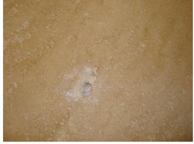
Above is a worst case scenario of the filler in a slab of Travertine coming loose / popping out. This is usually caused by poor fitting or weak travertine (Commercial Grade), but all Travertine is subject to the filler coming loose due to the nature of the material.
